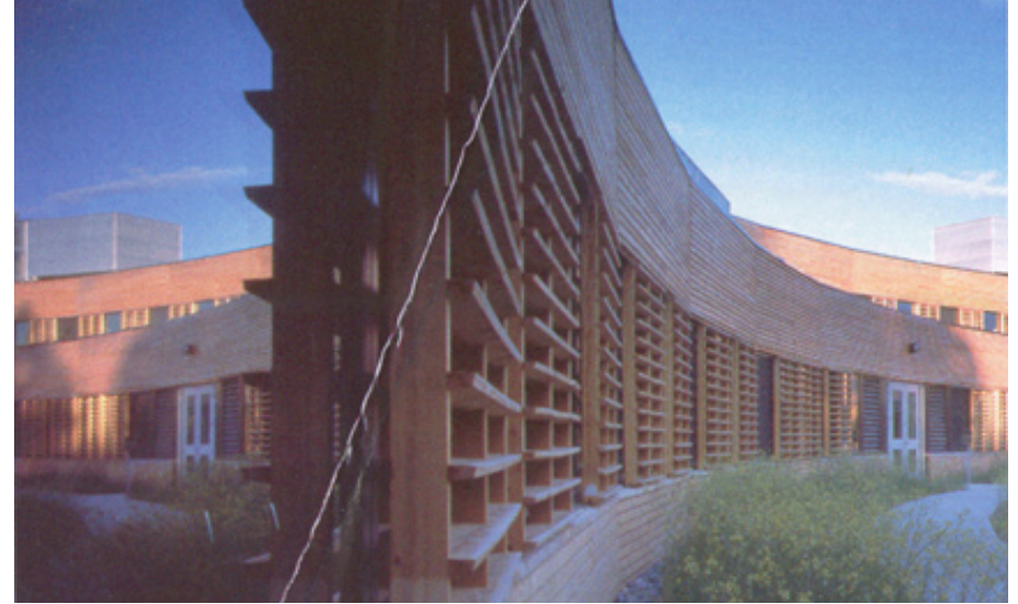
Figures 11 and 12: Detail views of the yellow cedar rain screen on the exterior.
