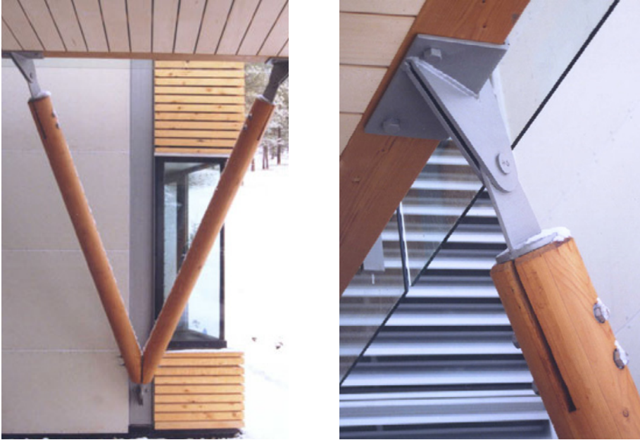
Figures 13 and 14: Detail views of the building's wood column connections.
