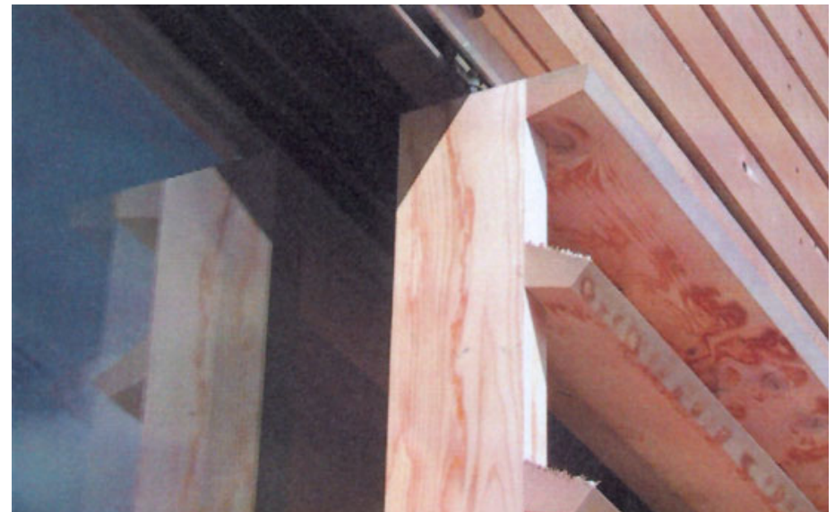
Figures 11 and 12: Detail views of the yellow cedar rain screen on the exterior.
